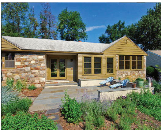
The final results of Diane Menke's holistic renovation show beautifully in this photo. Design assistance by In House Studio, LLC. Photo by D. Landry
